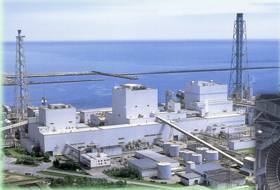
Tomatoh-Atsuma Thermal Power Station (Courtesy of Hokkaido Electric Power Co., Inc.)
